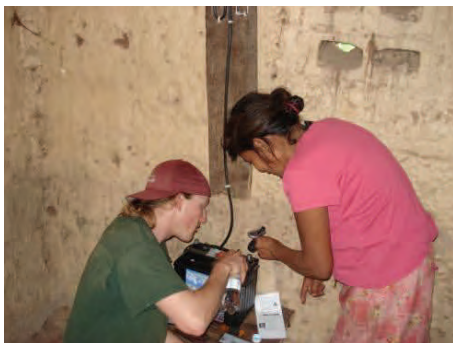
Figure 14. John showing her how to fill battery with distilled water.
